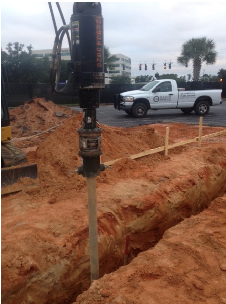
RS3500 Pipe Extension installation
