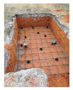
7" x 7" x 0.5" new construction pile caps to allow for connection to the new poured concrete footings.
