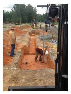
Anchor cap set seven (7) inches from bottom of footing (L).Extension bolted to lead section (R). Lead sections with 10",12",14" helices (Background). All CHANCE material is hot dipped galvanized for corrosion protection.
