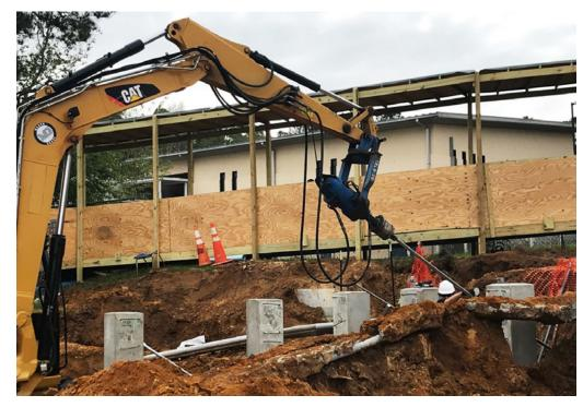
89 SS125, SS5, and SS150 Helical Tiebacks to secure concrete piles for new concrete retaining wall. 8-32-kip allowable capacities.
