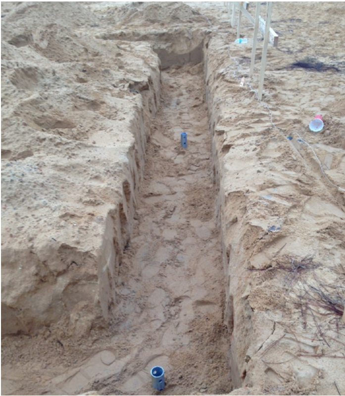
Top view of completed helical pile installation prior to installing the new construction cap.
