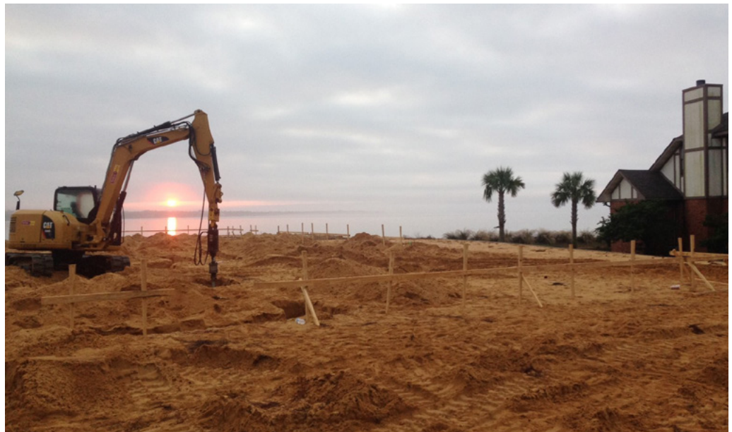
View of the work area in relation to adjacent structure.
